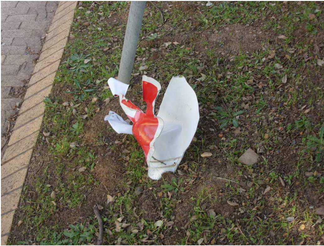
Figure 2 Damage caused to a road sign.
