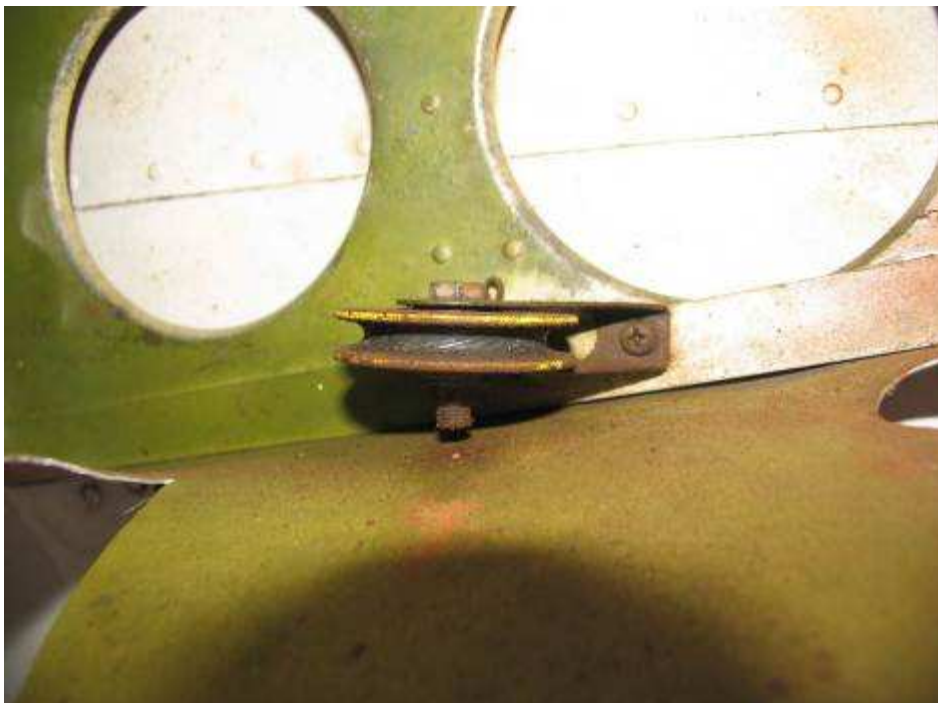
Figure 11. A close-up view of the pulley (Section B) that supports the right-hand rudder cable
