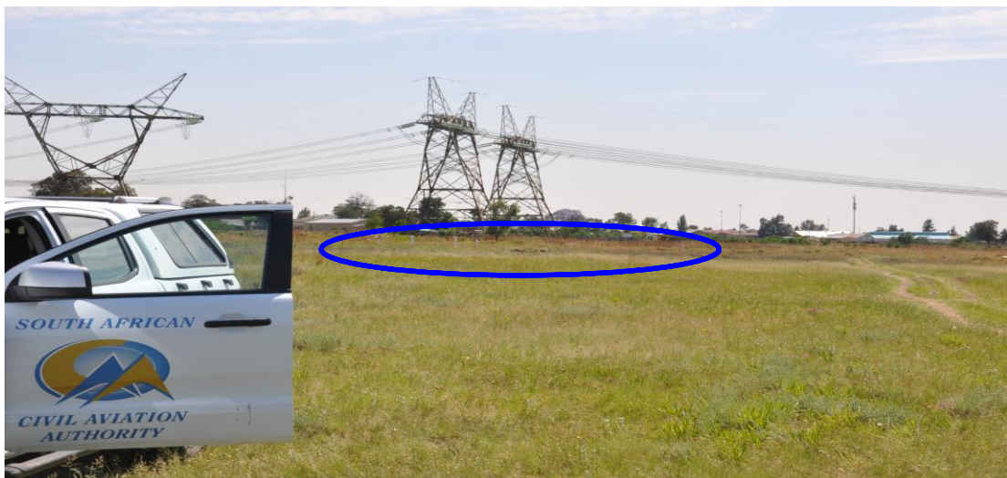
Figure 18: Obstacles and construction rubbish dump towards the end of the field
